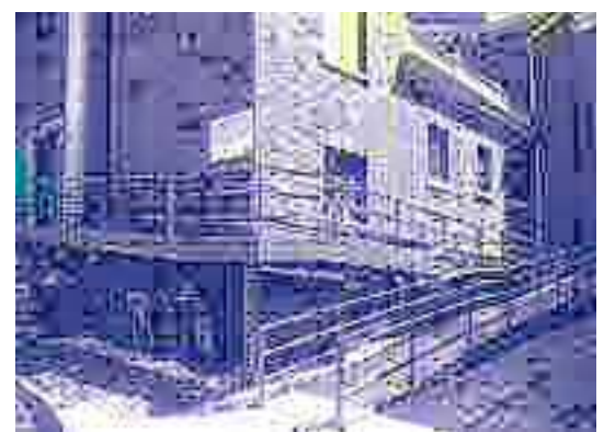
Figure 6: This ramp is too long, is too steep, requires frequent maintenance (painted steel) and has an industrial appearance. Neal Vogel for Restoric, LLC
