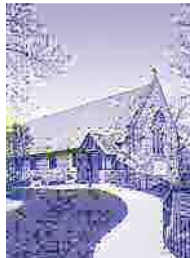
Figure 5: At this entrance, a small stoop was replaced with a bermed walk and landscaping to create accessibility. Neal Vogel for Restoric, LLC
