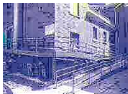
Figure 6: This ramp is too long, is too steep, requires frequent maintenance (painted steel) and has an industrial appearance. Neal Vogel for Restoric, LLC
